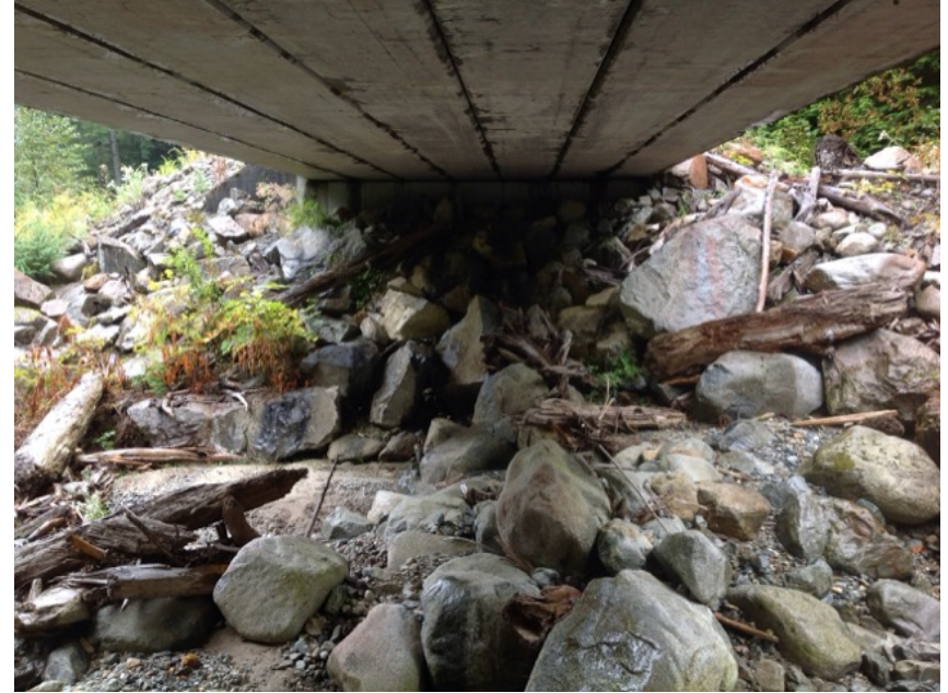
Right Bank Abutment when facing downstream
