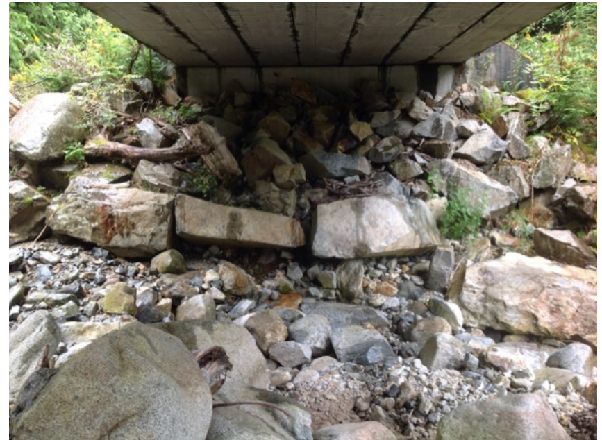
Left Bank Abutment when facing downstream
